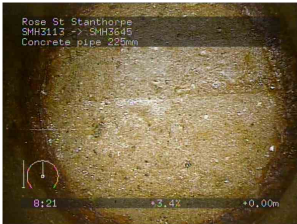
SMH3113 - SMH3645_0733ade3-9d6a-46ff-ad89-590ab6010539_202004 27_082230_162.jpg, 00:00:00, 0.00 Start node, maintenance hole, Nodename:, SMH3645
