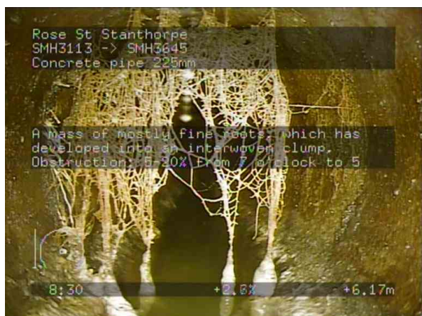
SMH3113 - SMH3645_a09c4ef3-edee-4f3a-b582-7686910014e3_20200427_083117_125.jpg, 00:05:59, 6.17 A mass of mostly fine roots, which has developed into an interwoven clump, Obstruction: 5-20% from 7 o'clock to 5 o'clock
