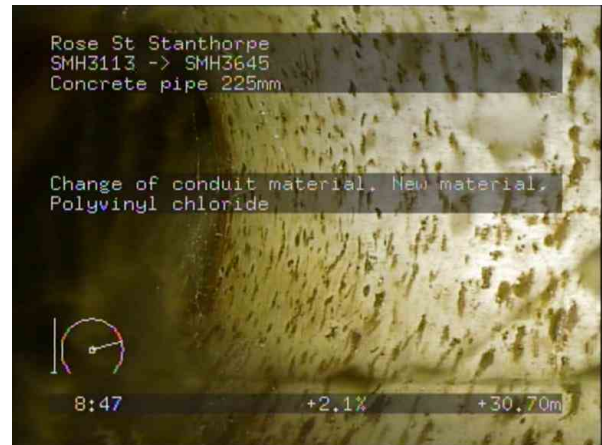
SMH3113 - SMH3645_55560e68-babf-4255-b72c-89af9cc7b23d_20200427_084823_820.jpg, 00:18:59, 30.70 Change of conduit material. New material, Polyvinyl chloride
