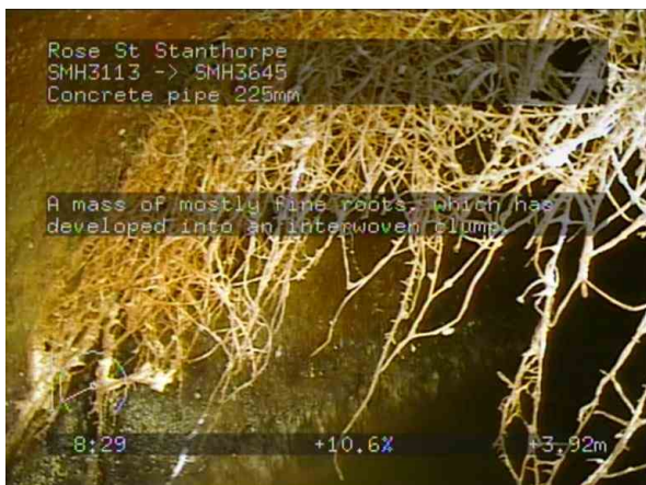
SMH3113 - SMH3645_b44c6d7d-2b95-45ce-ba5c-b1e081f2c3c1_20200427_083004_935.jpg, 00:04:57, 3.92 A mass of mostly fine roots, which has developed into an interwoven clump, Obstruction: 5-20% from 8 o'clock to 4 o'clock
