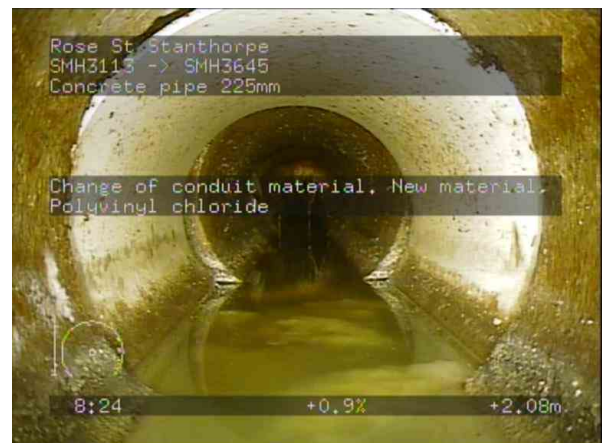
SMH3113 - SMH3645_eb0aba98-0190-4a3f-87af-436d8ab76472_202004 27_082459_238.jpg, 00:02:32, 2.08 Change of conduit material. New material, Polyvinyl chloride
